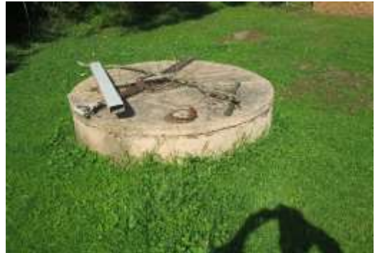
Figure 8 - reinforced concrete septic tank along the eastern site boundary of 484 Bringelly Road.
